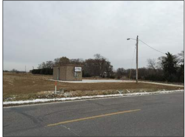
Photo #14 Utility building on west side of the Property.
