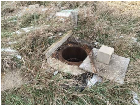
Photo #23 Abandoned water well.
