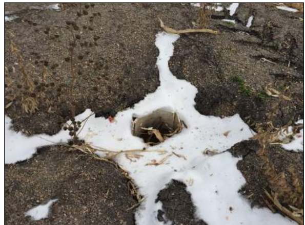
Photo #24 Abandoned water well.
