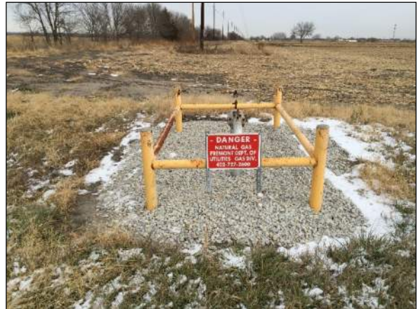
Photo #22 Natural gas pipeline, crossing the north side of the Property.
