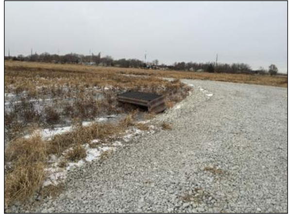
Photo #20 Trash located in the middle of the Property.
